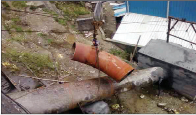
Reducing Bend being placed in position
