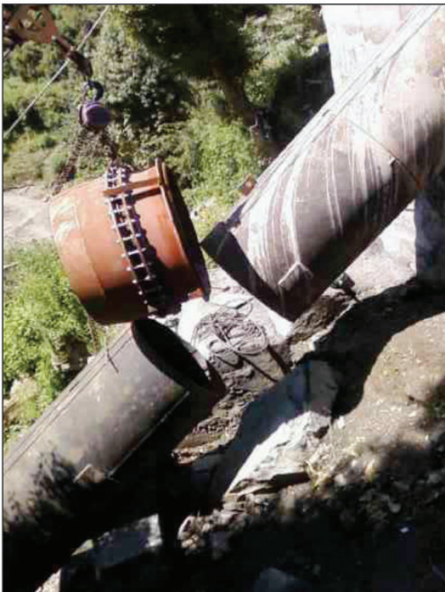
Expansion Joint being placed in position
