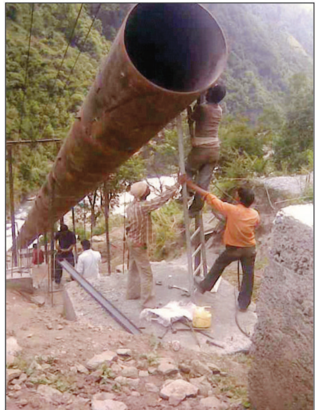
Penstock Erection in progress
