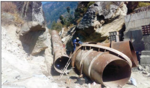
Bifurcation Pipe being welded at site
